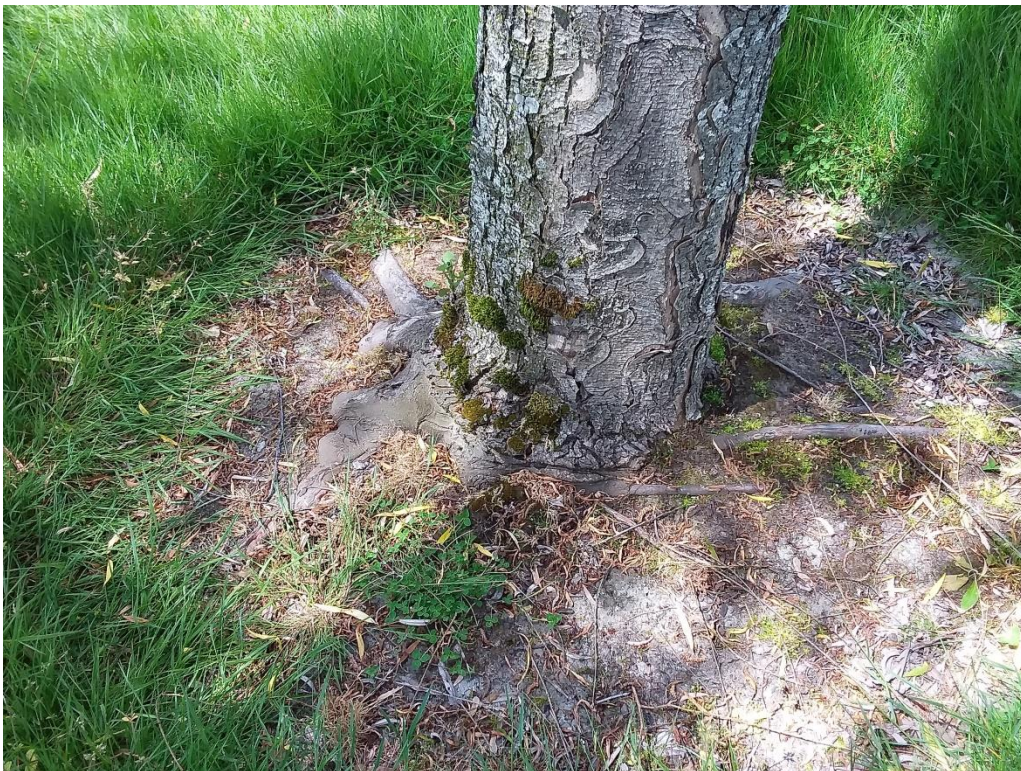
Figure 16. Looking at the base of the #10 maple.
