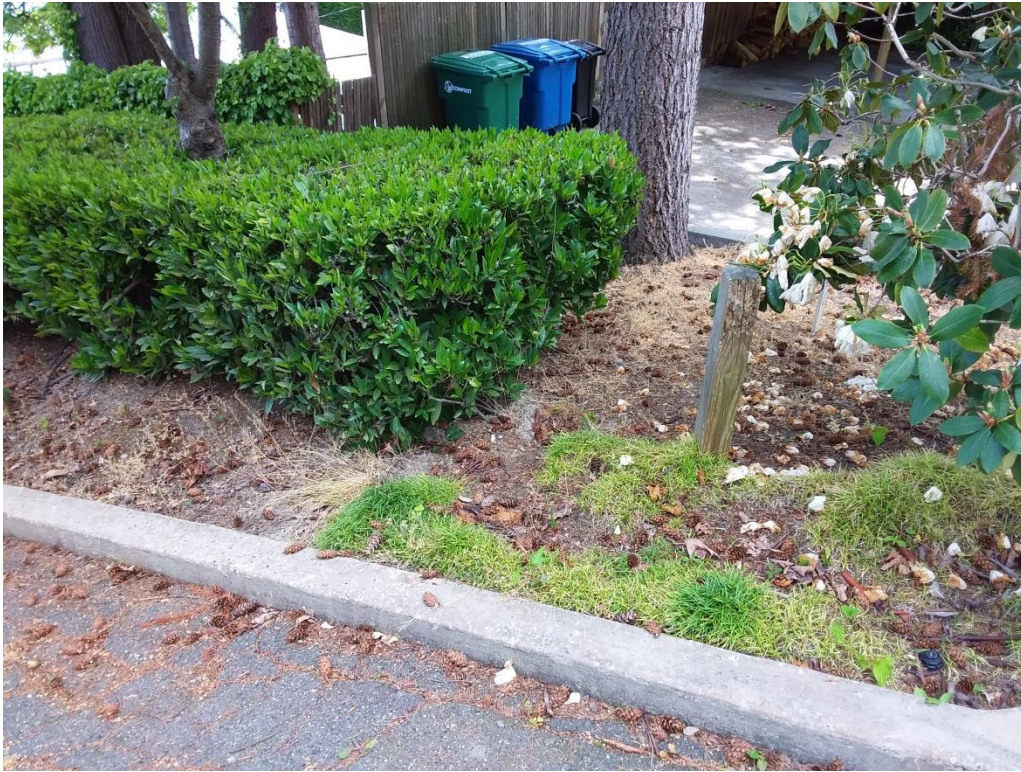
Figure 31. Looking south at the base of the #16 tree showing subject curbing. It is only 11.5' away at the point.
